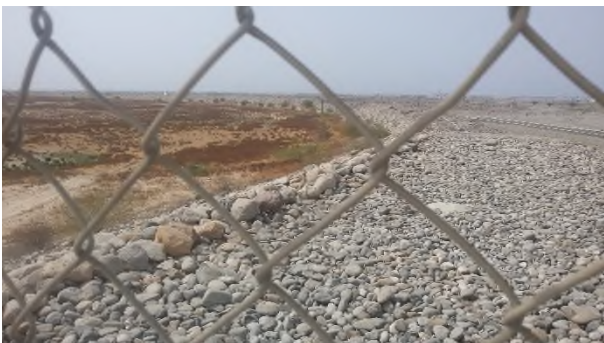
Figure 3: Al Khoud Recharge Dam, Oman, upstream of dam with recharge zone for infiltration of storm water runoff
