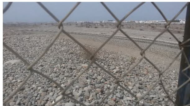
Figure 4: Al Khoud Recharge Dam, Oman, downstream of dam, recovery / emergency wells for public water supply
