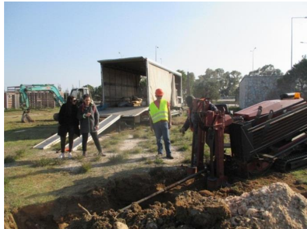
Figures 5. Horizontal Directional Drilling well
