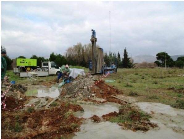
Figures 4. Drilling of the first side well
