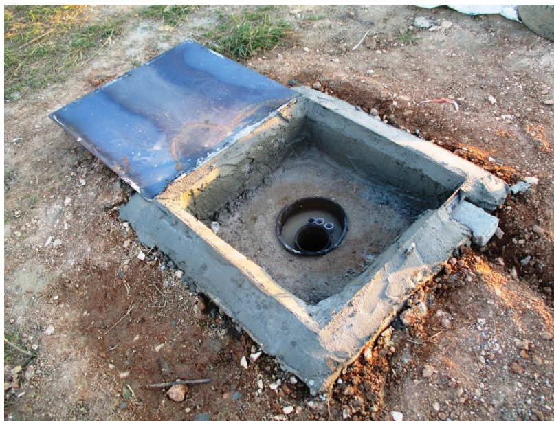
Figures 6. Installation of the reinjection point
